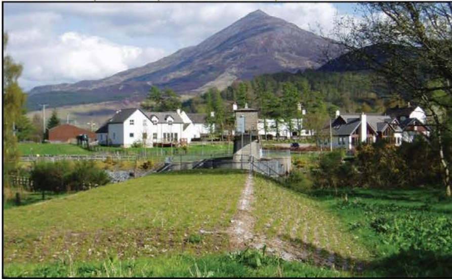
Photo 2 – Example of Completed Scheme using Voided Blocks
